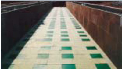
Figure 2: After installing the isolation (green)
