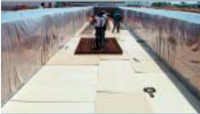
Figure 3: Block preparation for pouring the foundation
