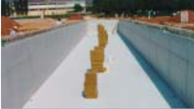
Figure 1: Foundation tank before installing the vibration isolation pads
